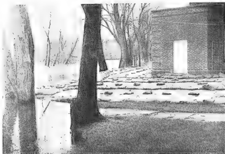
Figure 4.--Polyethylene and sandbags placed to protect loam and levee north of the Laboratory and Garage. Water level 15.4' on April 18, .4' below the April 20 crest of 15.8'. Photo taken by Bernard L. Berger.
